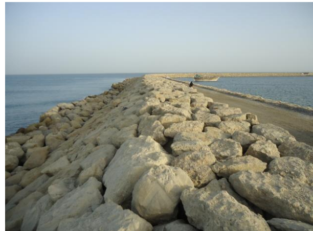
Figure 1. Bahal berm breakwater in the Oman Sea.
