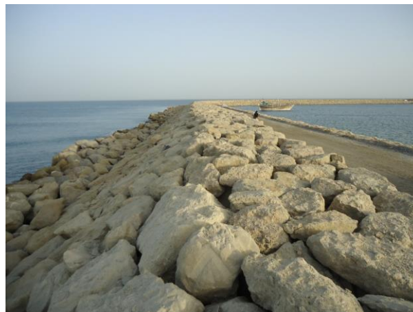
Figure 1. Bahal berm breakwater in the Oman Sea.
