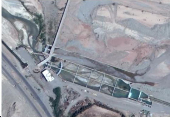
Figure 4. Aerial view of diversion dam in Garmsar.
