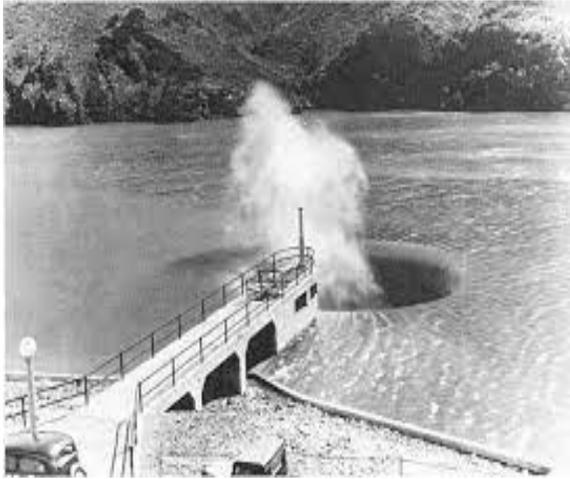
**Figure 4.** Piping phenomenon on shaft Morning Glory Spillway
