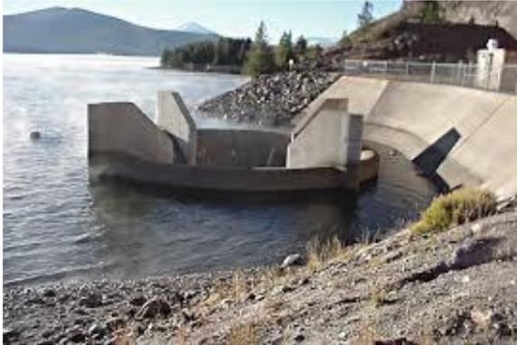
**Figure 2.** Anti-vortex blades on crest spillway
